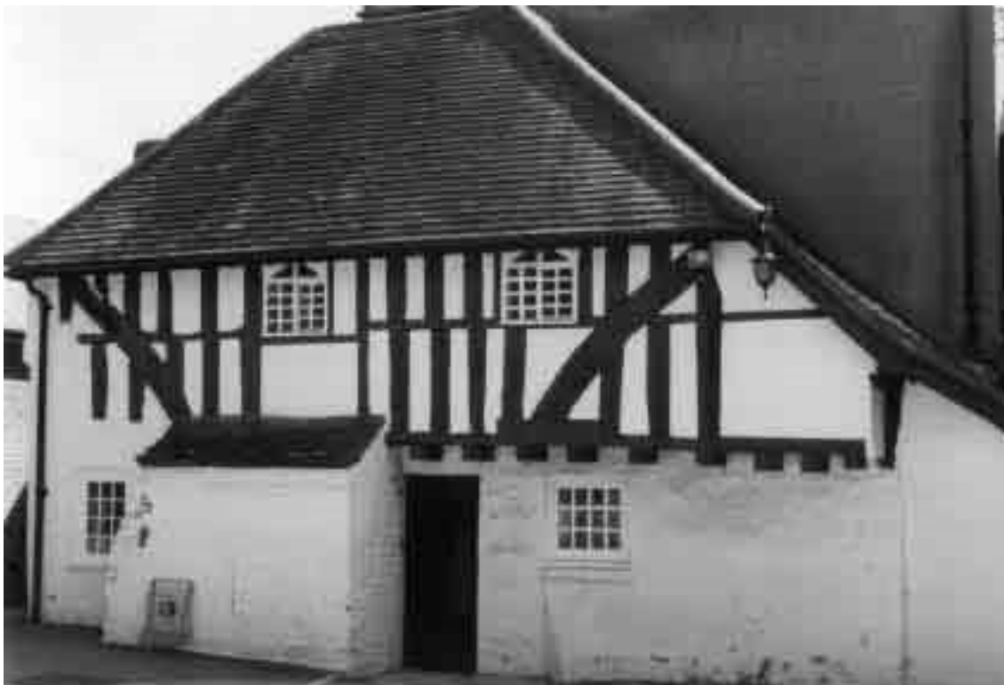
The timber framed cottage. Part of the old Moulsecomb manor house and one of the oldest buildings in Brighton
